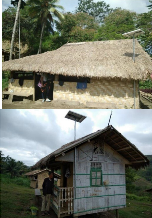
Diagram 8: Roof-through Pole mounted installations on thatched roof
