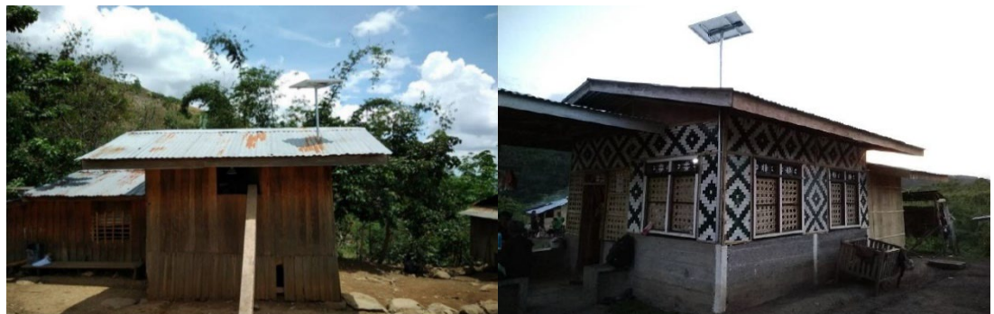
Diagram 7: Roof-through Pole mounted installations on GI roofs
